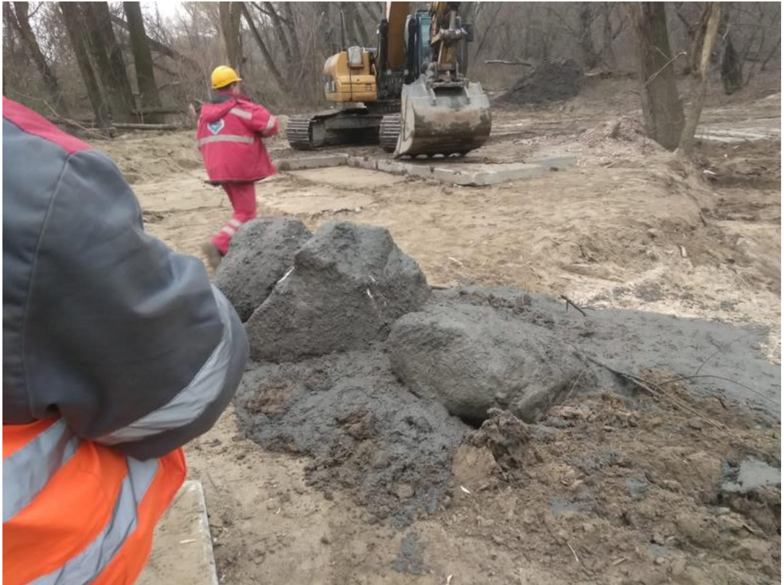
glacial boulders pushed into the final chamber and partially worn away by the cutting head
