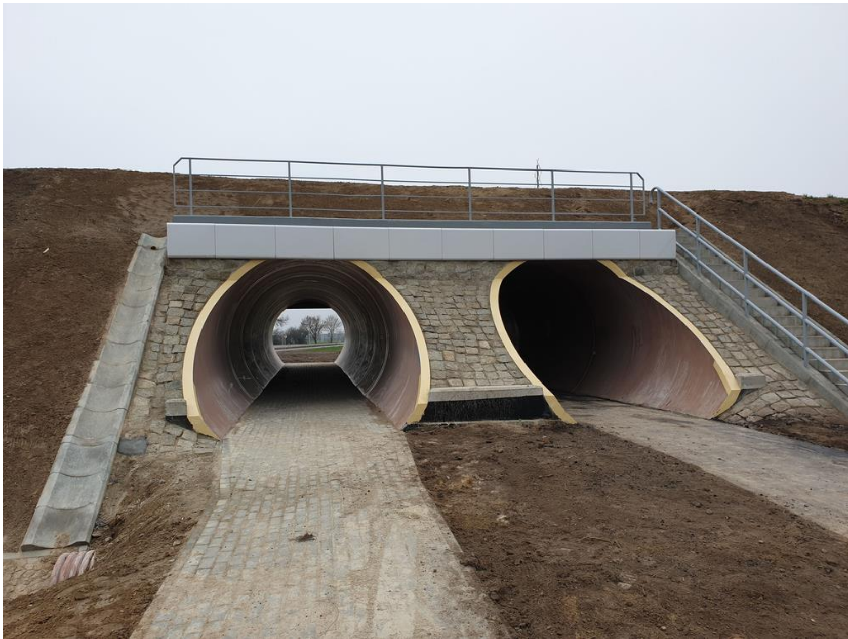
underpass for pedestrians and cyclists, Parczew, 2019
