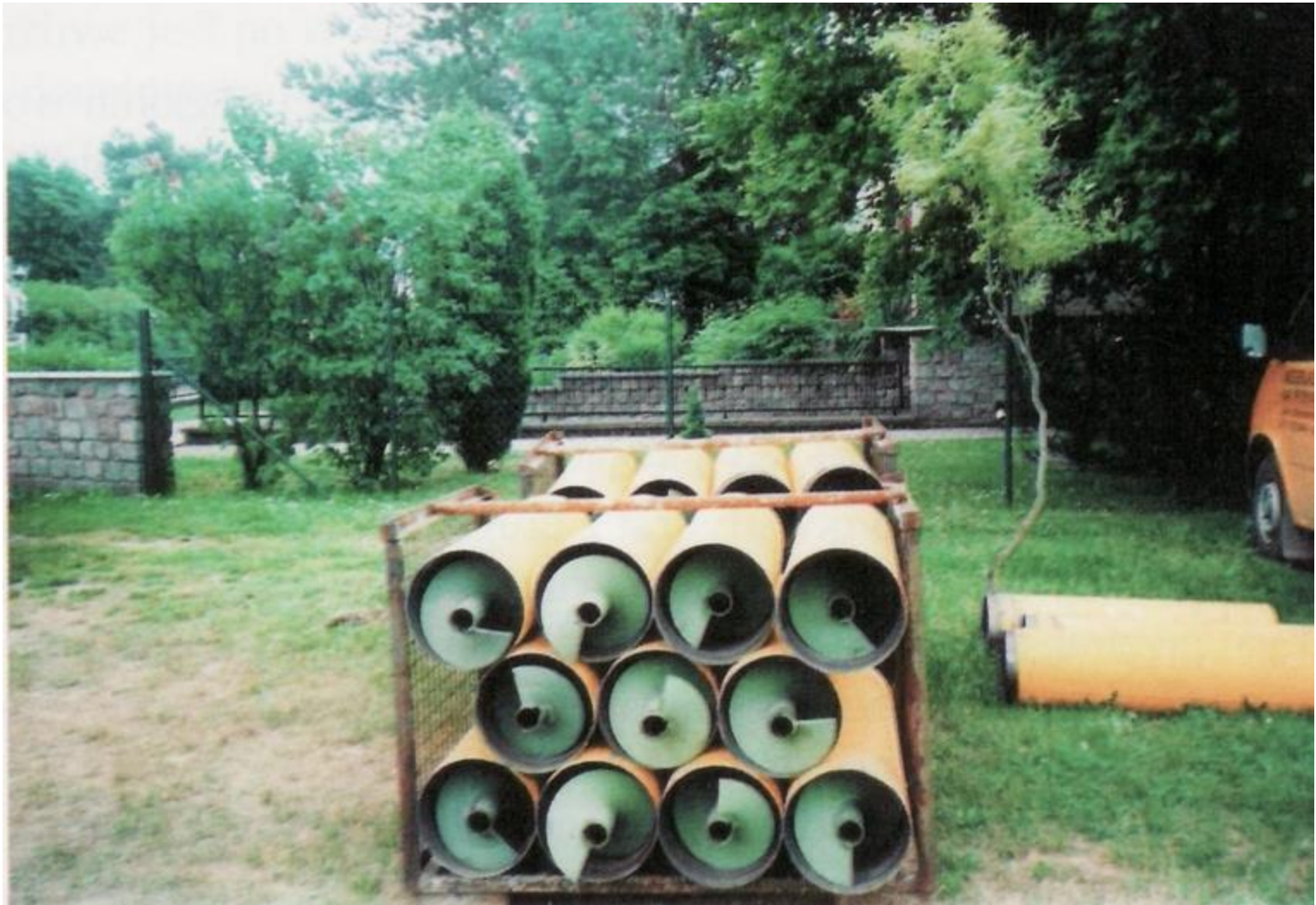
a set of steel casing pipes with the appropriate elements (parts) of the auger conveyor
