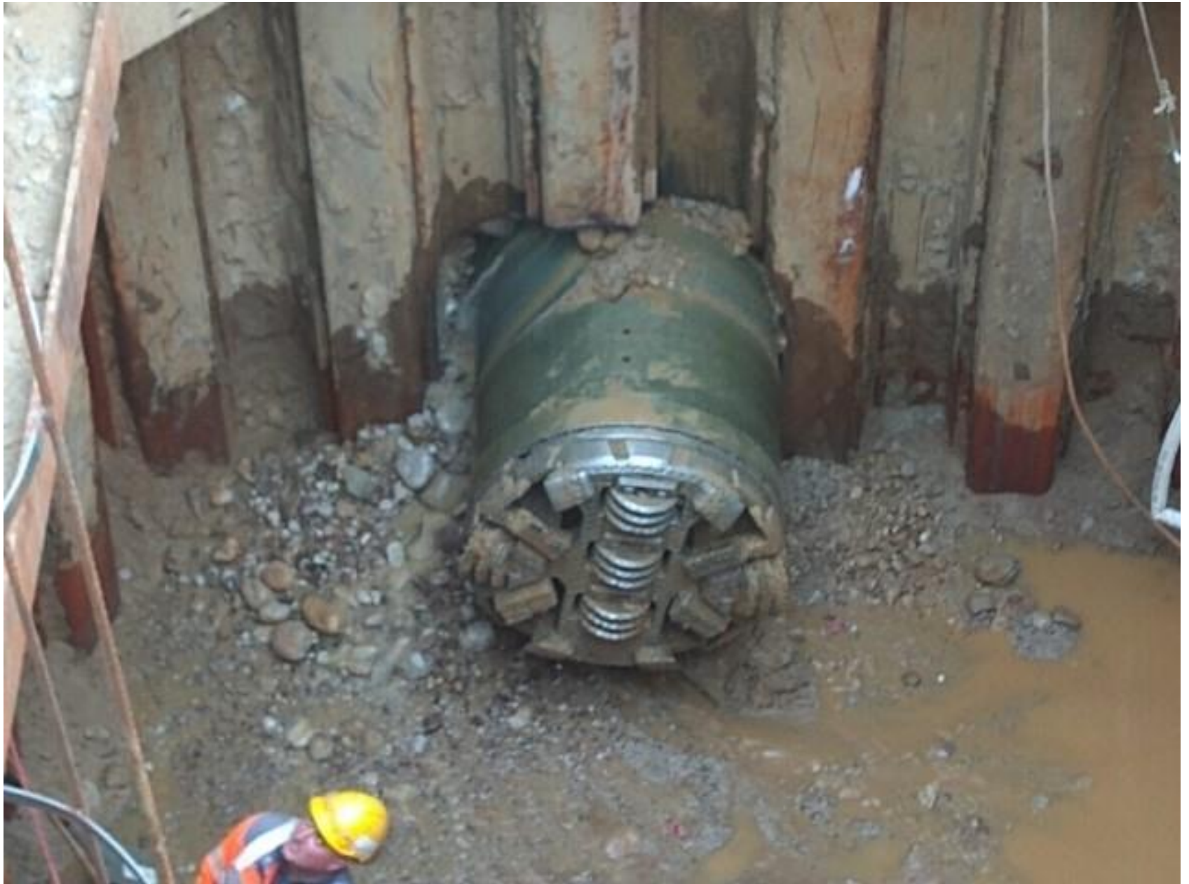
heavily worn ground-excavating disc
