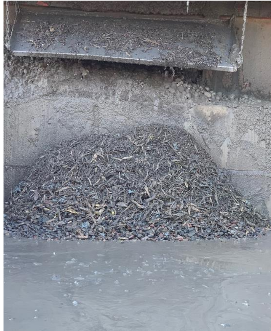
cut chips of tree trunks lying in river sediments – as an obstacle overcome by head of microtunneling machine.
